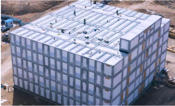
Ulanqab Huawei Cloud Data Center
